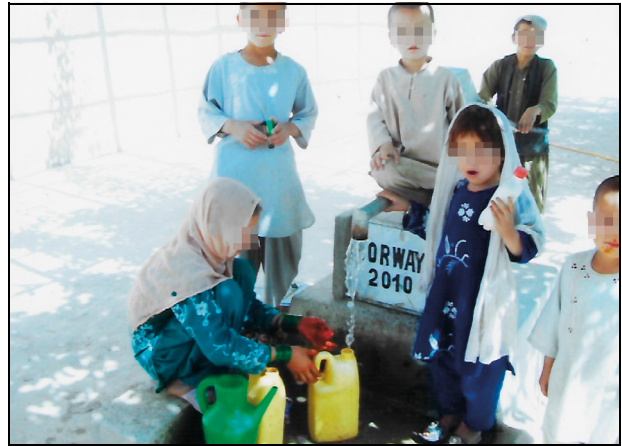
Figure 9.1 Norway carried out some small-scale aid projects in southern Afghanistan that were intended to benefit peace diplomacy efforts. This is one of about twenty wells that were constructed near Kandahar.
